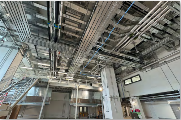
Electrical Installation at HASSC project
