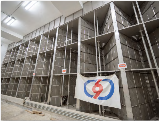
Air Purification System Plenums in the East and West Ventilation Buildings circulate fresh air and extract vehicle exhaust to maintain optimal air quality.
