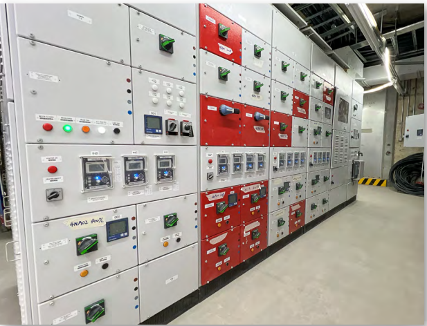
Low Voltage Switchboard at Kwu Tung Station Project
